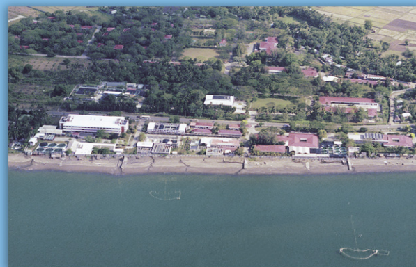
Tigbauan Main Station
