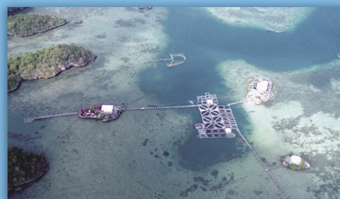
Igang Marine Substation
