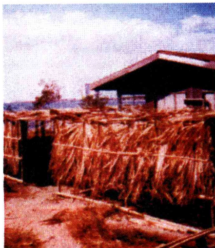
Mangrove nursery made up of bamboo poles with fish net and coconut fronds as roofing material
