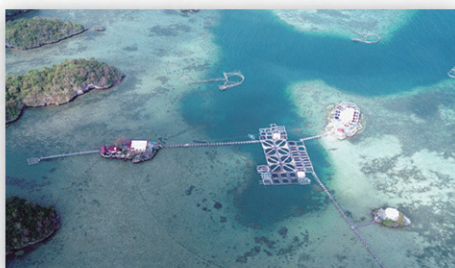
Igang Marine Substation
