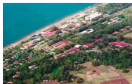
Tigbauan Main Station
