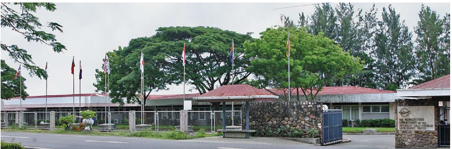
Tigbauan Main Station
