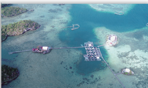
Igang Marine Substation
