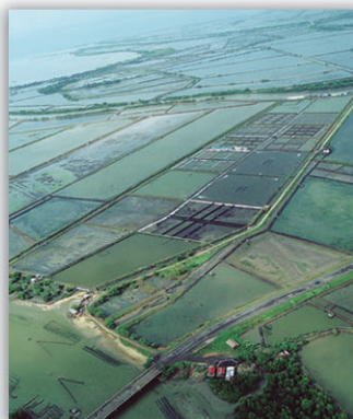
Dumangas Brackishwater Substation
