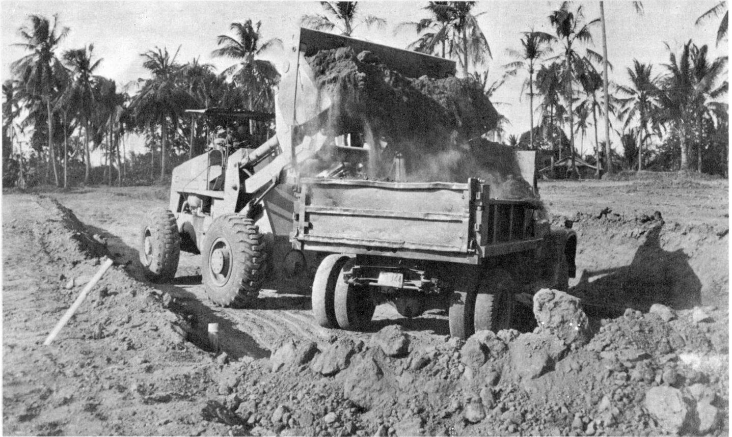
Construction of the internal road system
