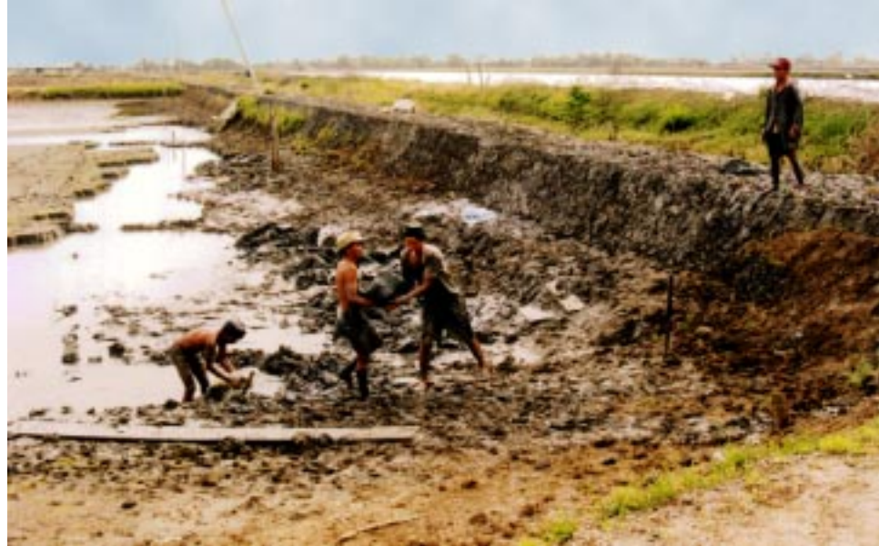
Contractual laborers excavating a pond.
