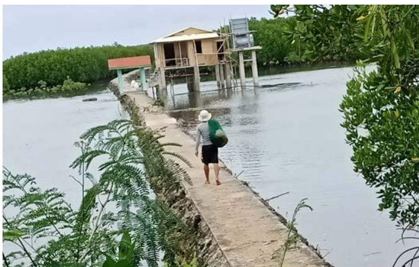
Abalone hatchery on stilts in nearshore buffer area at Sagay Marine Reserve due to lack of access to land, similar to the social constraints of marginalized fisherfolks
