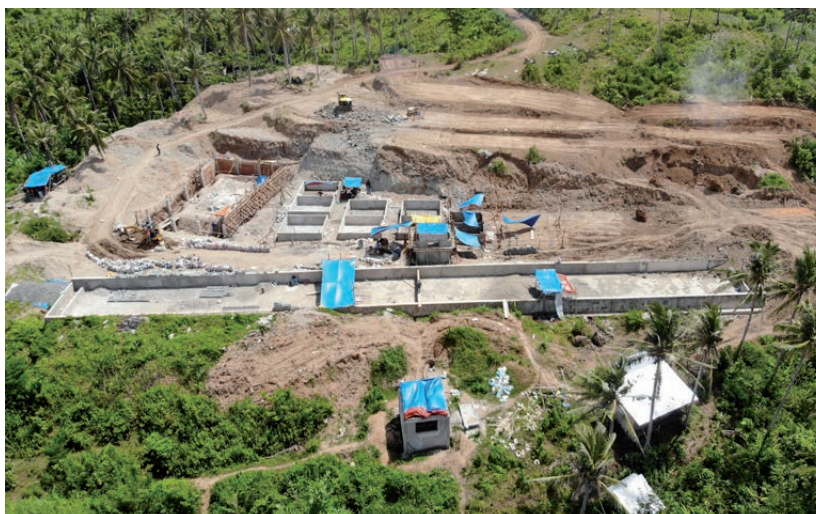
Multi-species freshwater hatchery under construction in Jabonga, Agusan del Norte
