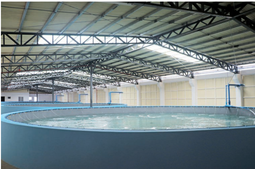
Inside the new Black Tiger Shrimp Broodstock Facility at the Tigbauan Main Station
