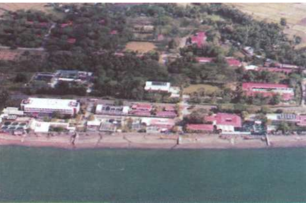
Tigbauan Main Station
