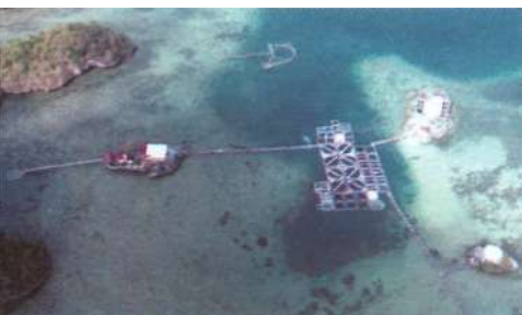
Igang Marine Substation
