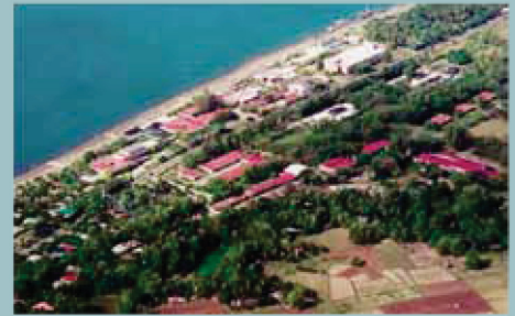
Tigbauan Main Station
