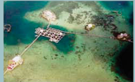
Igang Marine Station
