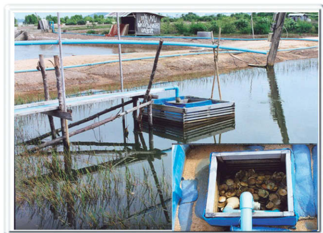
Fig 3. Sand filter box as a physical filtration in the treatment pond
