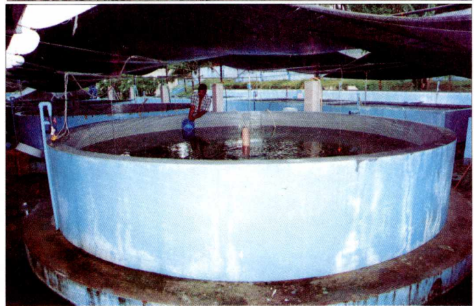
The Integrated Fish Hatchery Development Complex at SEAFDEC/AQD's Tigbauan Main Station (top), and a 20-ton circular larval rearing tank inside the complex
