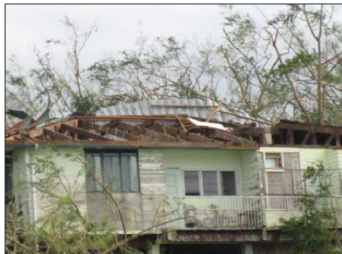
Roof of duplex C got blown off
