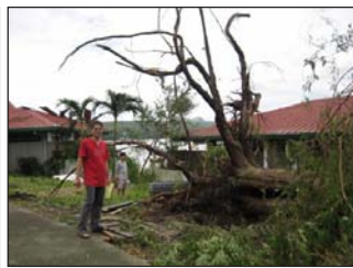
Downed transformers and electric post amidst the blown-off roof of the Generator House
