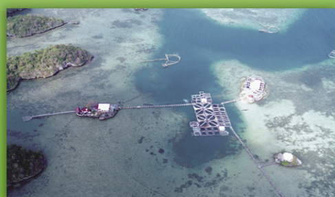
Igang Marine Substation
