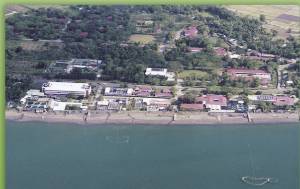
Tigbauan Main Station
