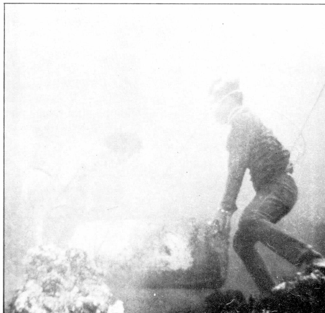
Fig. 5. Divers manually hauling the reef block.
