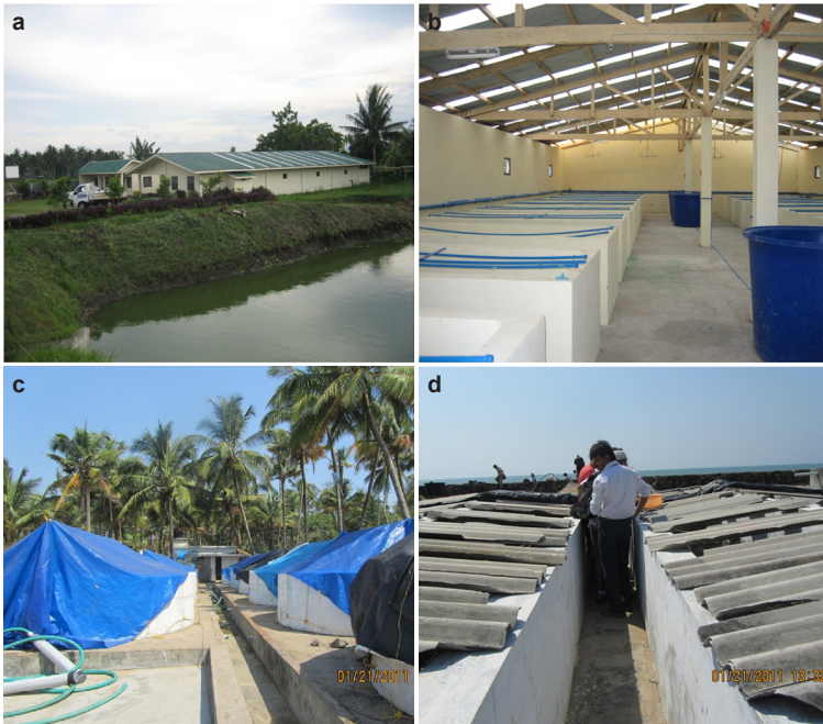
Fig. 19. Indoor (a&b) and outdoor (c&d) freshwater prawn hatchery facilities. The roof is provided with skylight for natural lighting in the indoor facility. The tanks may be covered with canvas or other materials to protect the outdoor tanks from intense sun and inclement weather.
