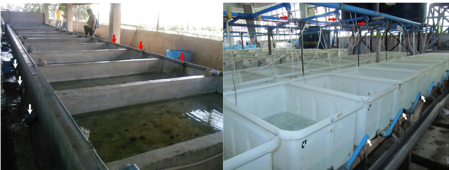
Fig. 22. Flow through system in concrete (left) and polyethylene (right) tanks. Red arrows show the inlet and white arrows the outlet for both systems.
