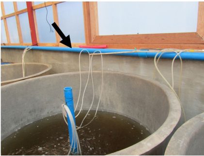
Fig. 28. Aeration fittings (black arrow) and aeration pump supplying oxygen to the tanks.
