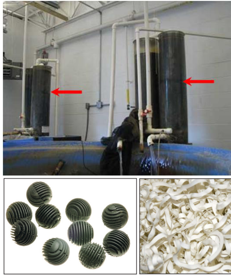
Fig. 21. Biological filters may be packed with materials which will provide good surface area (bottom photos) for the growth of beneficial microbes to remove nitrogenous wastes.
