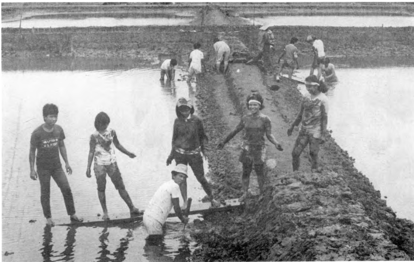
Trainees constructing ponds
