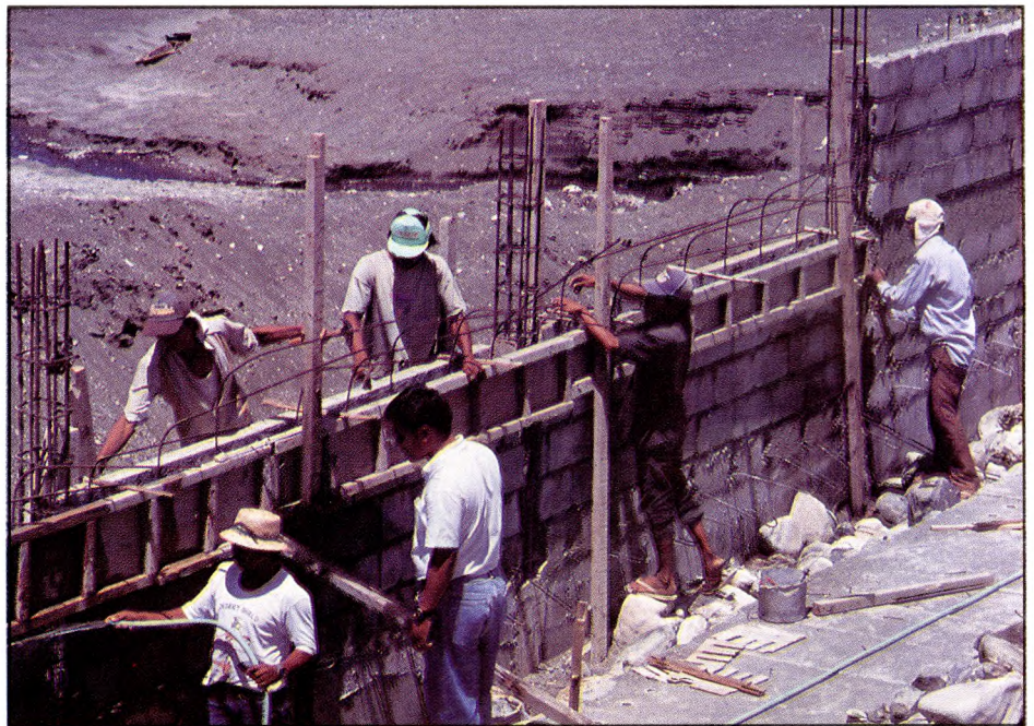
A perimeter fence was started on the seaward side.
