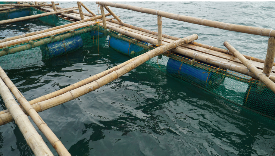
Figure 3. Bamboo divisions to accommodate 2 m x 2 m nursery net cages
