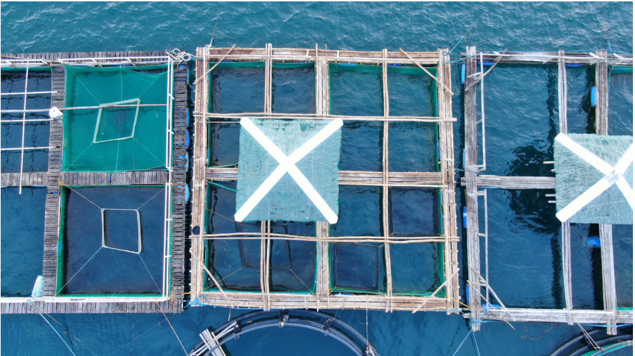
Figure 2. A 10 m x 10 m modular cage divided into four compartments - 5 m x 5 m grow-out cages or 16 compartments - 2 m x 2 m nursery cages
