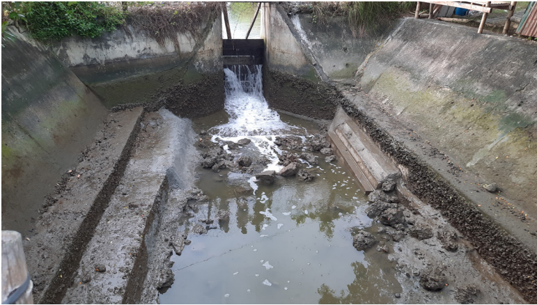
Figure 4. Clearing of debris in canals to provide efficient drainage system
