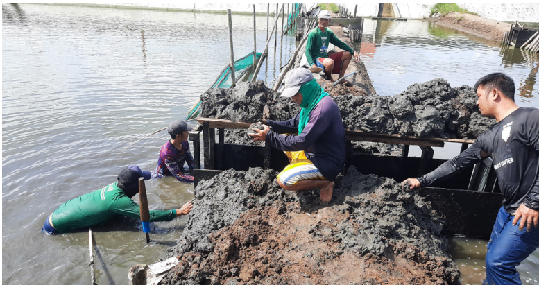
Figure 5. Repair of pond gates and dikes to prevent water seepage
