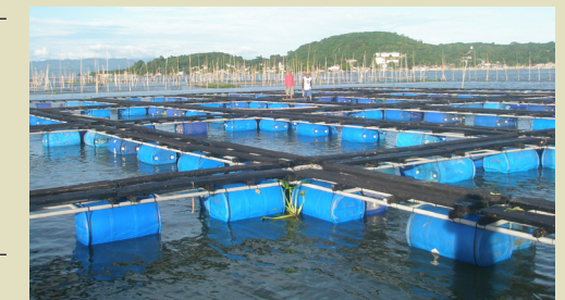
Floating cage module with plastic drums as floats
