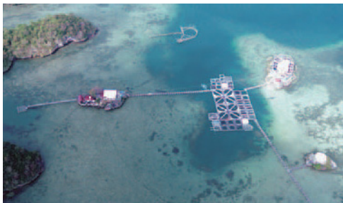
Igang Marine Substation
