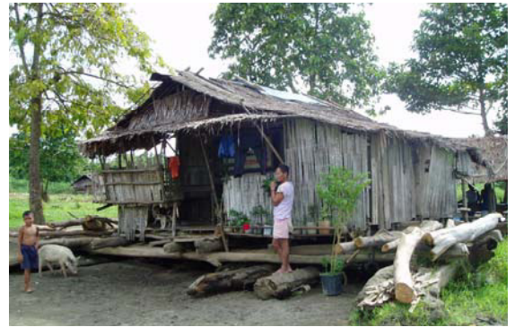
To survive the regular flooding, houses in the Marsh must be able to float. (above)..... or be on high stilts (below)
