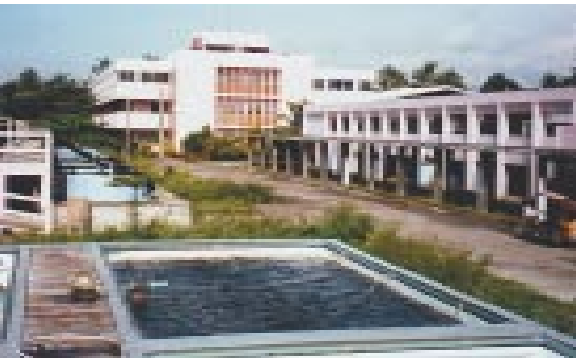
Tigbauan Main Station
