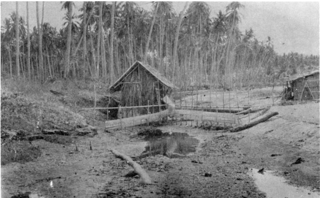
Fig. 16. Tidal set net with matted bamboo wings set in small tidal creek (Dinaig, Maguindanao).
