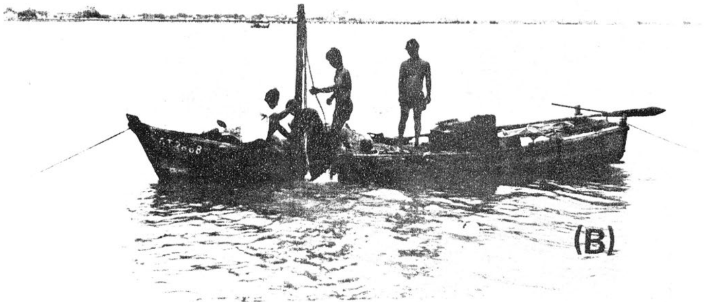
Fig. 4. (A) A wooden peg used to anchor the floating net-cages in Penang. (B) The fishermen use the weight of the boat to drive the peg into the bottom soil. The metal chain is attached to a pulley system.
