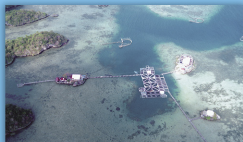
Igang Marine Substation
