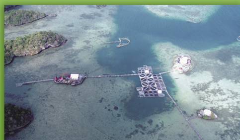
Igang Marine Substation
