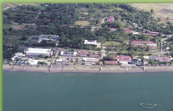
Tigbauan Main Station
