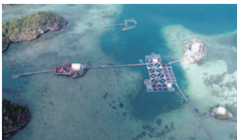
Igang Marine Substation
