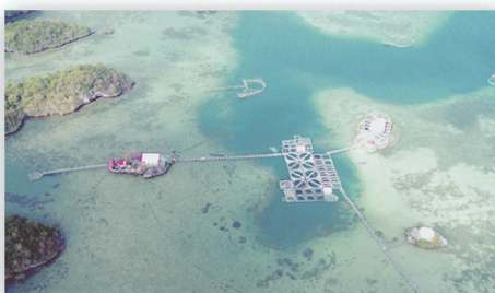
Igang Marine Substation
