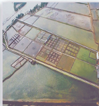
Dumangas Brackishwater Substation
