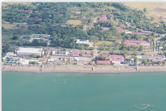
Tigbauan Main Station
