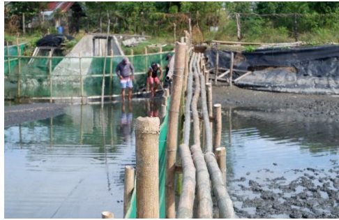
Figure 6. Bamboo bridge construction
