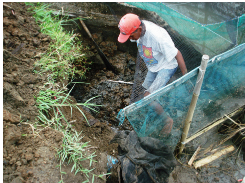
Figure 23. Repair of leakages and seepages in the dike near the gate
