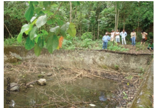
Top: Dr. MJHL Ramos and Dr. EG Ayson get their feet wet when their dump truck got stuck in the middle of the river. Above: One of the assessed sites with an existing concrete compartment
