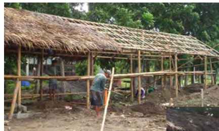
On-going construction of the Marine fish and abalone backyard hatchery
