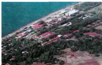
Tigbauan Main Station
