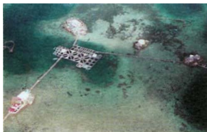
Igang marine Substation
