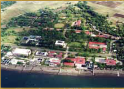
Tigbauan Main Station (TMS)
