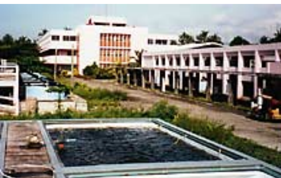
Tigbauan Main Station
