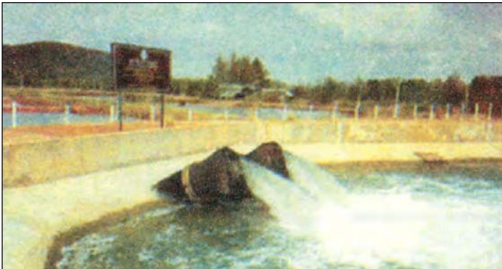
Seawater released (below, left) to main canal for the shrimp ponds (right)
